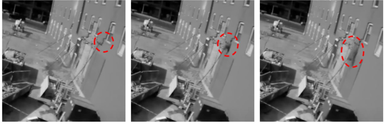
44. Approximately 44 seconds before the catastrophic collapse more bricks from the area previously identified as imminently hazardous fell away.
